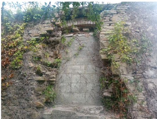
Plate 15: Blocked up school window in exterior of wall. Looking east
