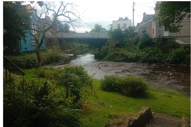
Plate 4: Tullow Bridge over the Mulkear. Viewed from the riverbank. Looking south
