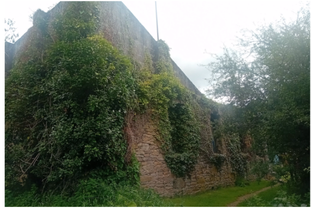
Plate 14: Extant west wall of school. Looking south-east
