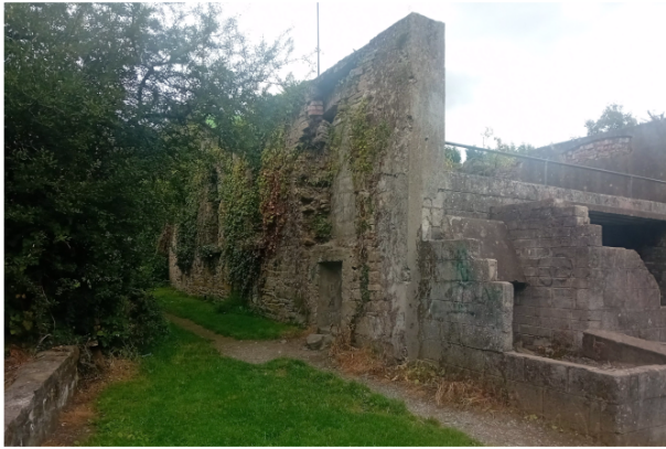
Plate 13: Extant west wall of western school, incorporated into handball alley. Looking north-east
